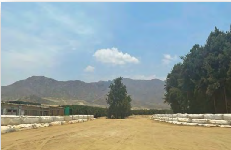
Geobags (retaining walls) are built around reservoirs and wells to protect them against potential damage caused by the flow of rainwater.
