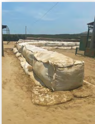
Geobags (retaining walls) are built around reservoirs and wells to protect them against potential damage caused by the flow of rainwater.
