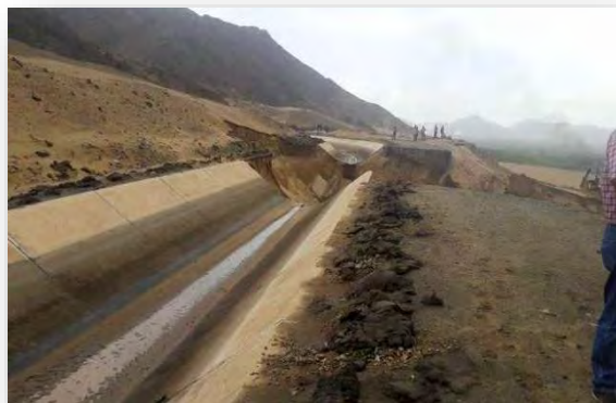
A landslide caused damage to a canal in the Chavimochic Irrigation Project in La Libertad in 2017. (Source: El Comercio )
