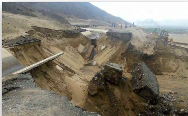
A landslide caused damage to a canal in the Chavimochic Irrigation Project in La Libertad in 2017. (Source: El Comercio )
