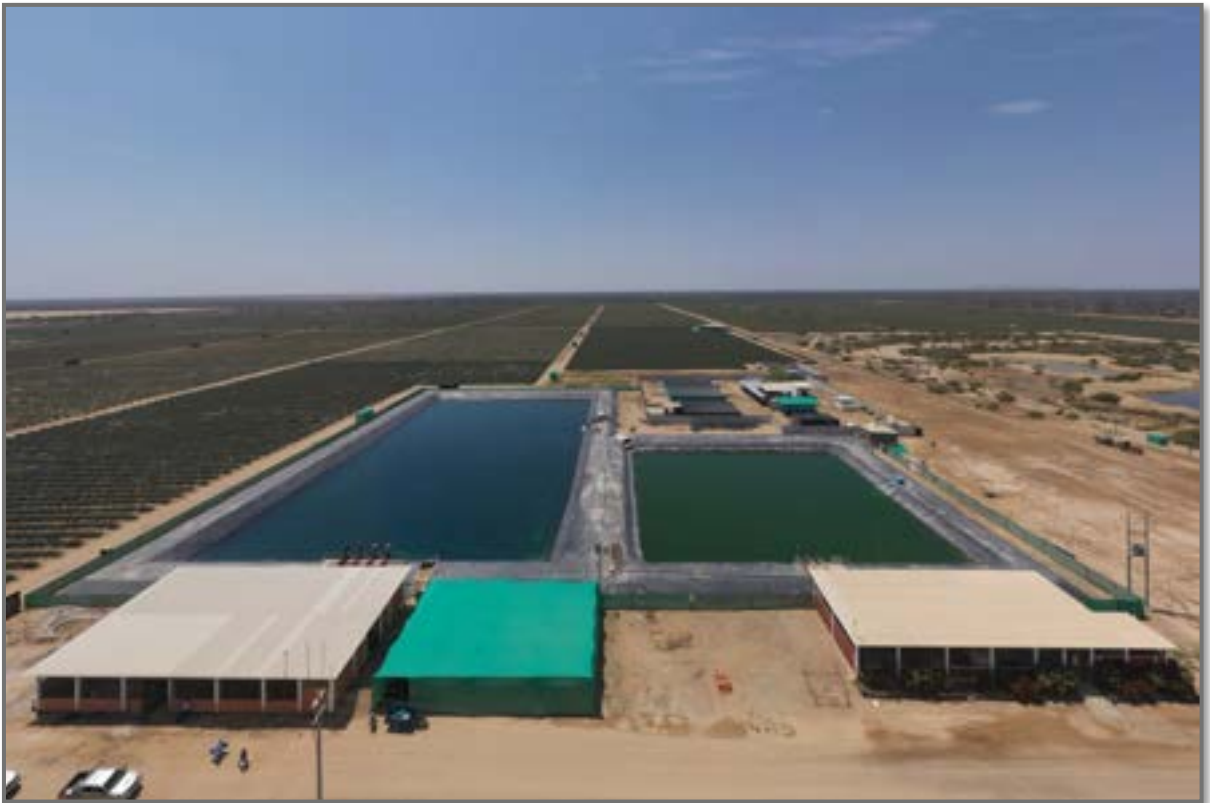
Jayanca (Lambayeque Region) water holding reservoirs, irrigation and fertigation system, and Osmosis System. Photo: supplied by Beta.
