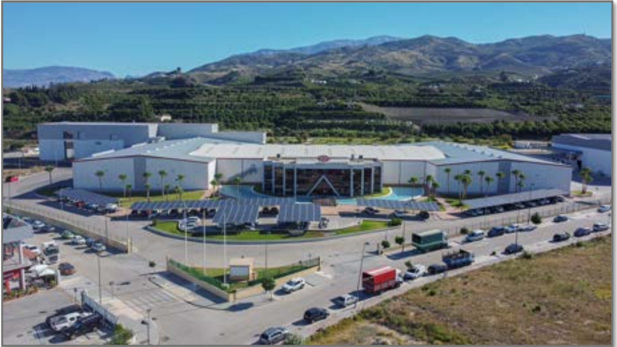
TROPS' headquarters in Vélez-Málaga. Photo supplied by TROPS
