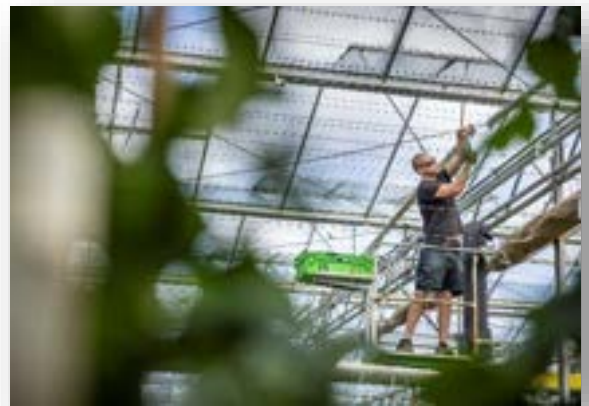
Thermal screens are being installed at the Geraghty glasshouse in Tūākau, New Zealand to improve its energy performance.
