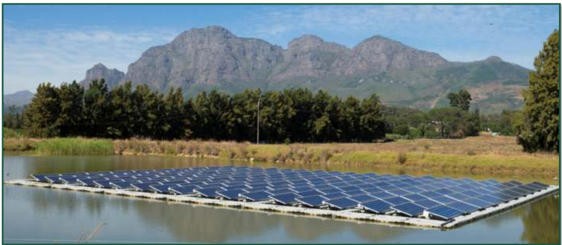
60 kW power floating solar. Photo: Carina Wessels
