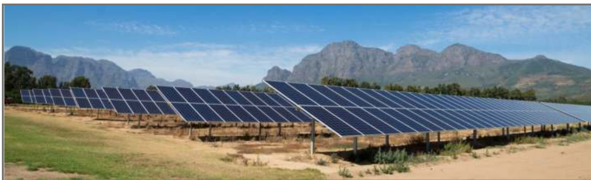
534 kW power ground mounted solar. Photo: Carina Wessels
